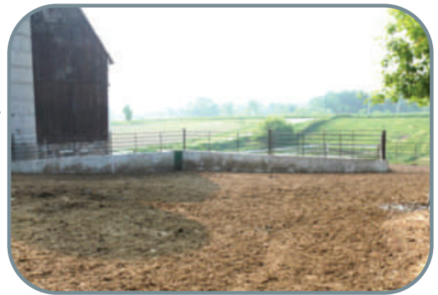
Figure 1: Barnyard with retaining wall that serves as temporary storage for runoff
