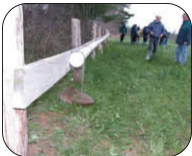
Figure 4: Distribution pipe with 1/2" holes at 17' intervals distribute runoff evenly across the strip
