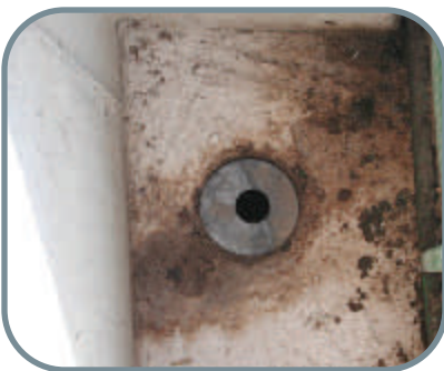
Figure 3: Properly sized orifice plate behind screen to control flow rate
