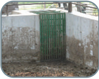
Figure 2: Three screens to minimize solids from being pumped to the strip
