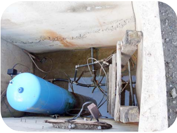
Photo 2. Well pit inside view
