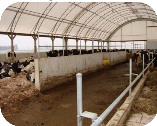
Photo 5: Interior of bedded pack dairy barn
