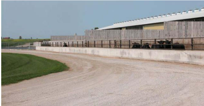
Figure 6. Barnyard with Interior Windbreak Partitions Which Minimize Wind Chill and Drafts.
