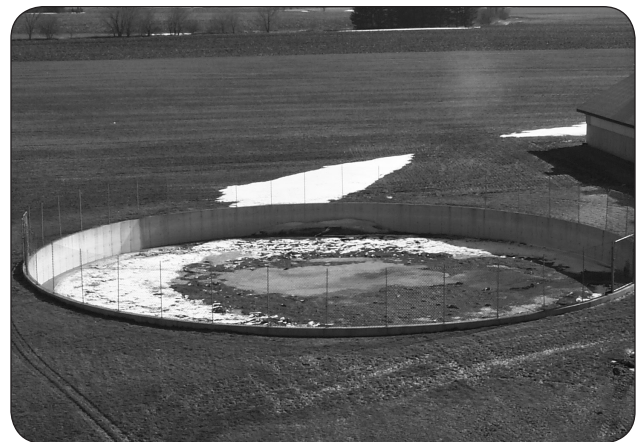
Figure 1. Open, circular, liquid tanks are commonly used on farms to store liquid nutrients such as manure from livestock operations.
