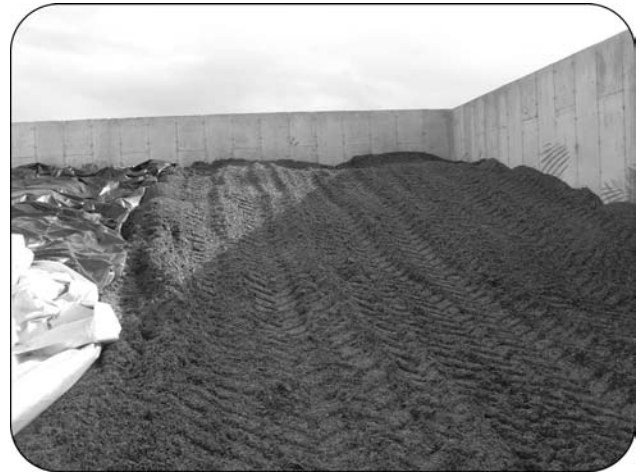
Figure 3. A horizontal concrete silo use to store drier off-farm materials such as corn husks and grape pumice.
