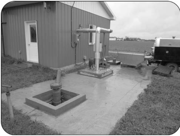
Figure 2. An in-ground co-substrate input tank where liquid off-farm materials such as fats, oils and grease are stored temporarily.
